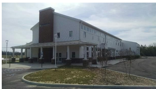
Figure 11 - Middle Peninsula Regional Transit Facility
